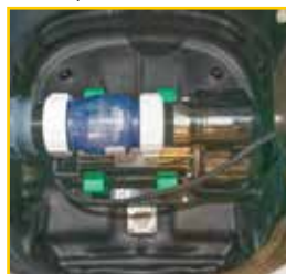
Check valve and sewage pump Mach II
